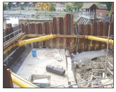
The work meant removing the old footbridge across the weir (the remaining half of the footbridge can be seen) and a temporary footbridge has been constructed. The whole job is a big project and when it is complete it will include a fishladder to allow fish to travel upstream past the weir.
